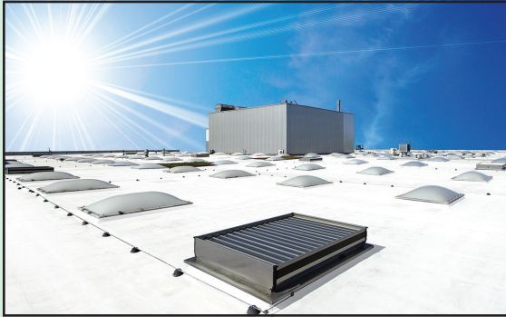
Kemperol Reflect 2K FR Cool Roofing system.
